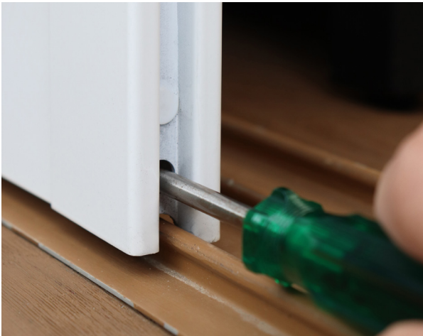
Adjust wheel kit to raise shutter and create clearance.
