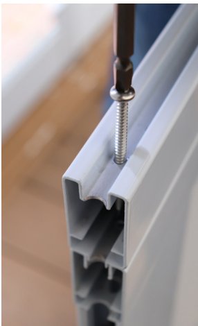
Fasten widener through pre-manufactured screw holes using supplied screws.
