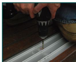
c. Secure lower track to the ground using appropriate screws.
