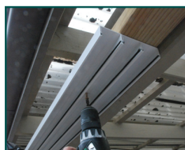
c. Attach upper channel to beam/spacer with wood screws.
