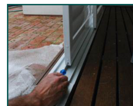
e. Adjust rollers until shutters move freely. Install track stoppers if required.
