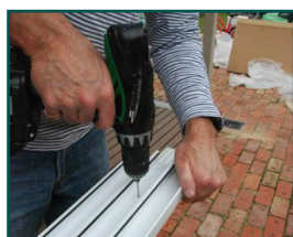
b. Pre-drill channel to allow wood screws to be inserted.
