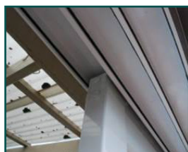
b. Centre of channel should be directly above the corresponding raised section on the lower track.
