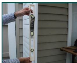
a. Using a level, locate the lower track directly below the upper channel.
