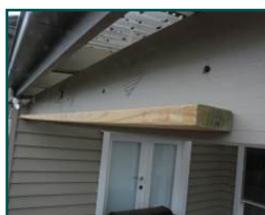
a. Fix spacer timber to top beam (if required).
